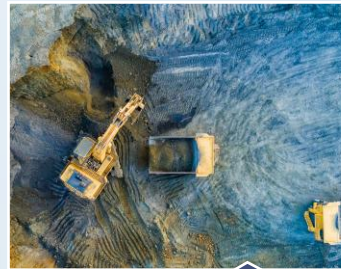
Metal Industry (metal surface treatment, mining, metallurgy)
