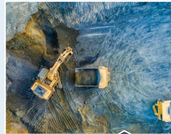
Metal Industry (metal surface treatment, mining, metallurgy)
